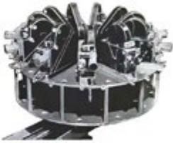
Above right is the mount and beam for the 16-millimeter Eastman Cine-Kodak Specials used to film Circarama
