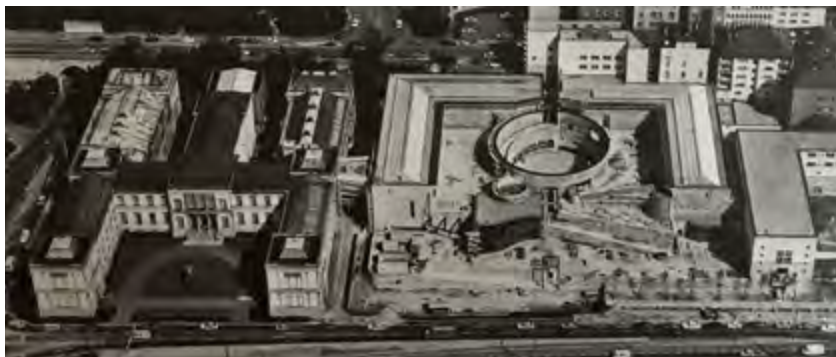
figura 8 Staadgalerie New Building and Chamber Theatre 1977/83. James Stirling y Michael Wilford, publicada en James Stirling, Buildings and Projects. Rizzoli, 1984
