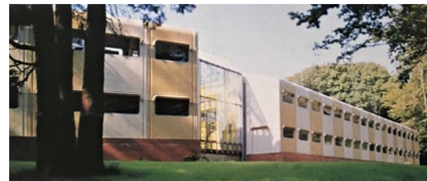
figura 7 Olivetti Training School 1969/73. Haslemere Surrey, R.U. James Stirling. © Richard Einzig, publicado en James Stirling, Buildings and Projects. Rizzoli, 1984
