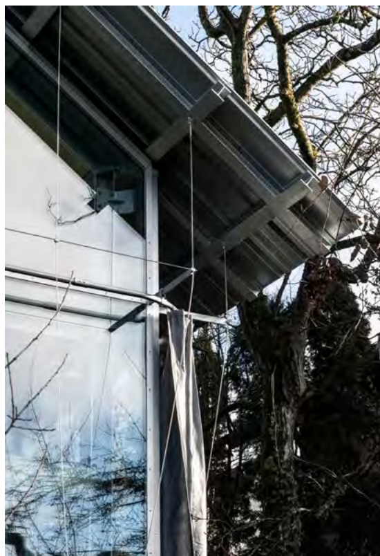
figura 5 Filter House, gentileza COMTE/MEUWLY
