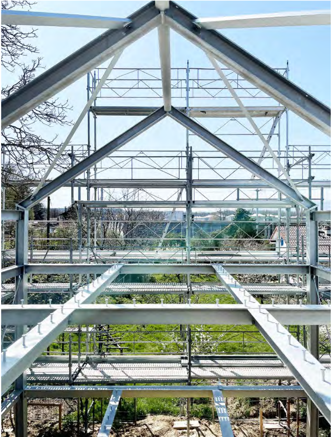
figura 2 Filter House, gentileza COMTE/MEUWLY
