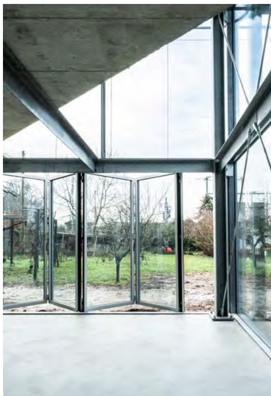
figura 4 Filter House, gentileza COMTE/MEUWLY
