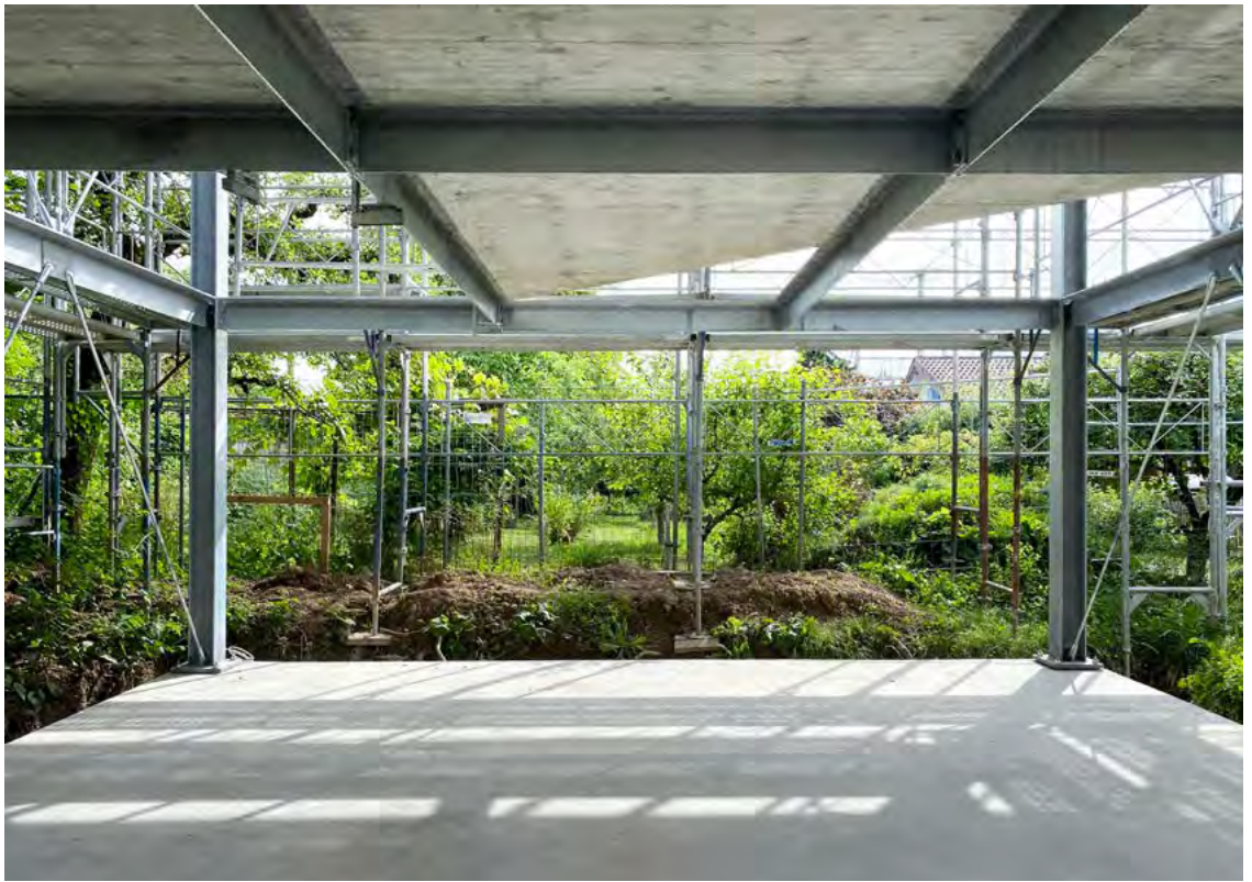
figura 3 Filter House, gentileza COMTE/MEUWLY
