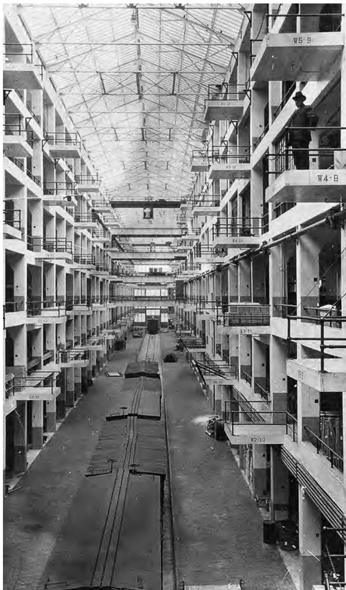
[5] Albert Kahn Inc. Fábrica Ford de Highland Park New shop. Vista interior. 1914. Prentz Family Archives.
